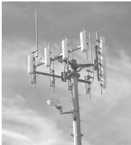
Figure 16.5 Sectorized base-station antenna.
